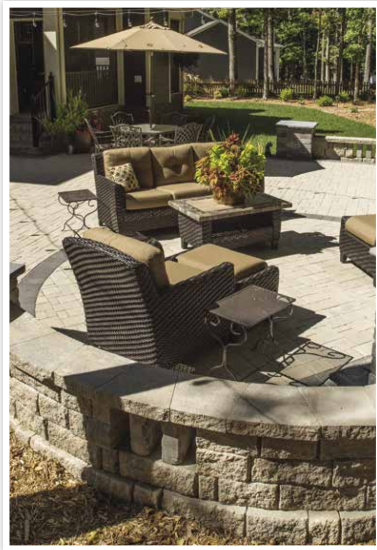
ABOVE: KingsLand Antiqued, Blue Ridge Color; Sitting Wall: Highland Stone® Freestanding, Blue Ridge Color; Sitting Wall Accent: Dublin™ Freestanding, Chesapeake Color; Wall Cap: Highland Stone® XL™ Cap, Bull Run Color; Column: Dublin™ Freestanding, Chesapeake Color; Column Cap: 32 x 32 Flat Rock Face Cap, Gray Color RIGHT: Sitting Wall: Highland Stone® Freestanding, Bull Run Color; Highland Stone® XL™ Cap, Bull Run Color
